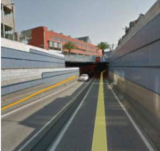
Figure 26. Street view of the exit from the tunnel.
