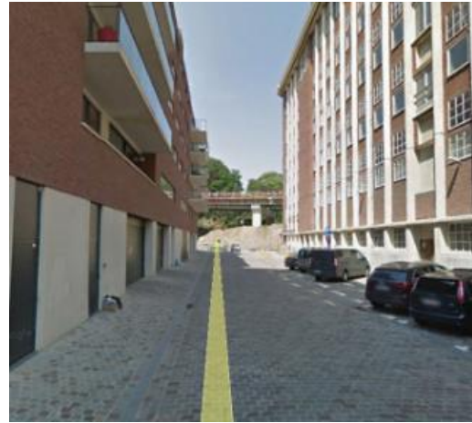
Figure 29. The street view of this ‘urban canyon’.
